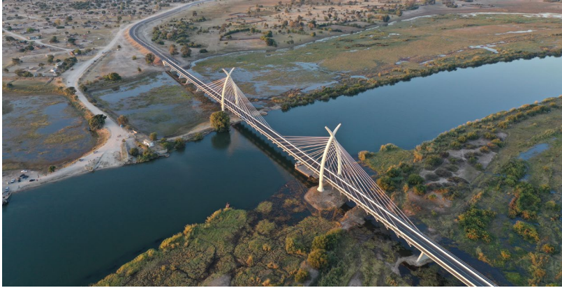
Client: Ministry of Transport & Communications - Roads Dept. Description: Construction of the cable-stayed bridge over the Okavango River - Botswana
