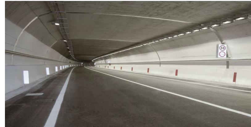
Client: Turin Agency 2006 Description: Construction of the Avigliana tunnel (tunnel 1.750 ml) - Avigliana (Turin)
