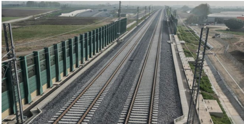
Client: CEPAV DUE Description: Construction of the railway connection HS/HC, stretch Treviglio-Brescia
