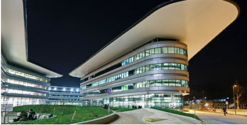
Client: University of Turin Description: Construction of New Einaudi Campus - Law School and Political Science - Turin
