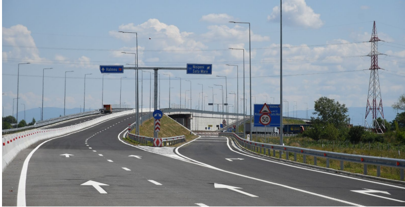
Client: C.A.L. C.N.A.I.R. S.A. Description: Satu Mare Bypass (Romania)
