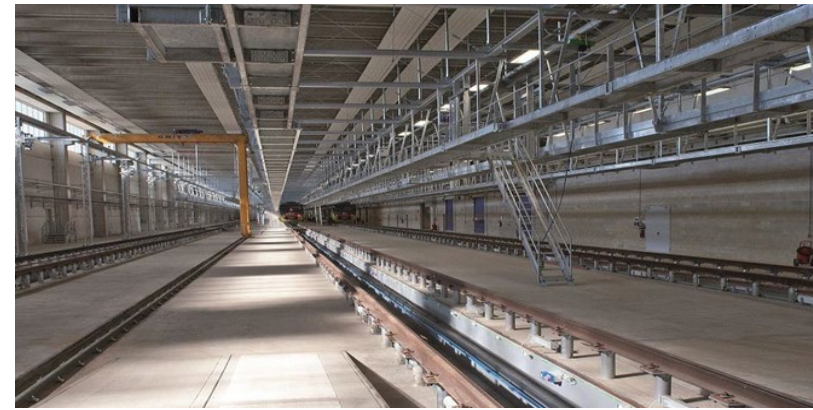
Client: Ferrovienord S.p.A. Description: Construction of the maintenance rolling stock plant in Camnago
