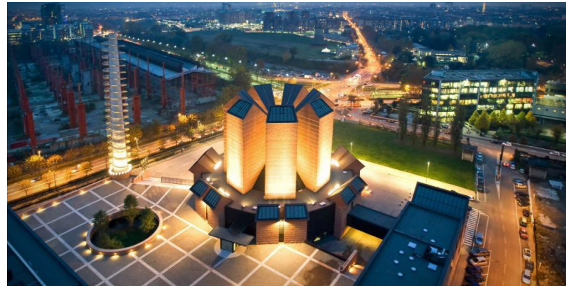
Client: Santo Volto Church Description: Construction Santo Volto Church - Turin
