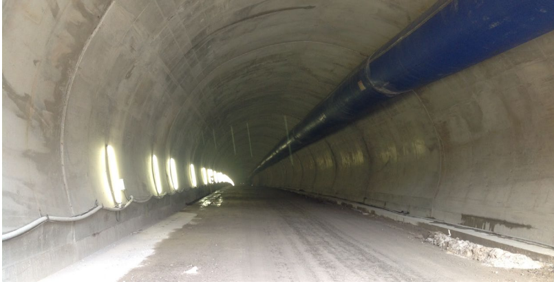
Client: Provincia di Bergamo Description: S.P. ex S.S. n. 470 (Province Road ex National Road n°470) Bypass to the town of Zogno (Bergamo)
