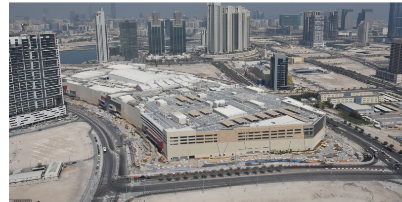
Client: AL FARWANIYA PROPERTY Description: Construction of the Abu Dhabi Reem Mall - UAE
