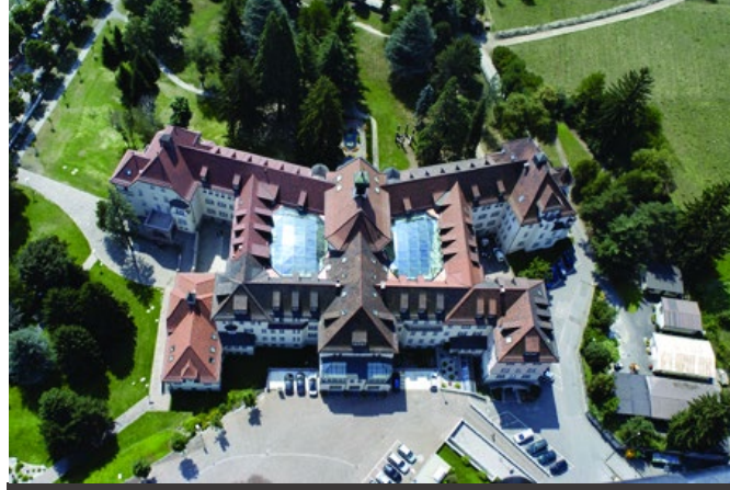
RENOVATION OF BRESSANONE HOSPITAL AZIENDA OSPEDALIERA BRESSANONE Bressanone (BZ)
