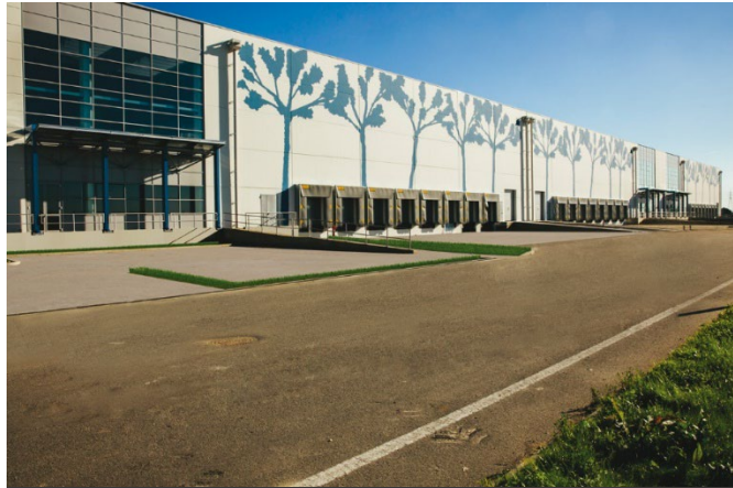
LOGISTIC BUILDING POLO LOGISTICO MORTARA SPA Mortara, PV
