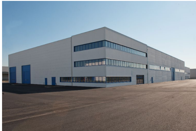
OFFICES AND LOGISTIC BUILDING SITO SPA Orbassano, TO
