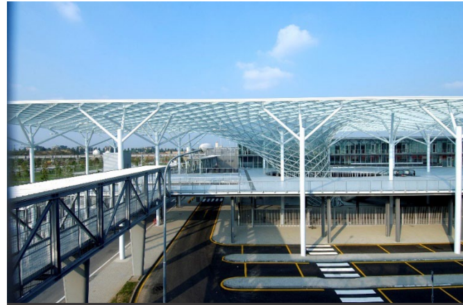
EXPANSION OF EXPO AREA IN MILAN AND CONSTRUCTION OF THE MULTISTOREY CAR PARK ENTE FIERA MILANO Milan
