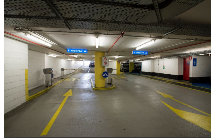
UNDERGROUND CAR PARK IN MEDA SQUARE PARCHEGGIO PIAZZA MEDA SRL Milan
